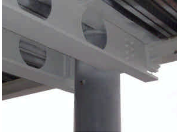
Tubular column connection
