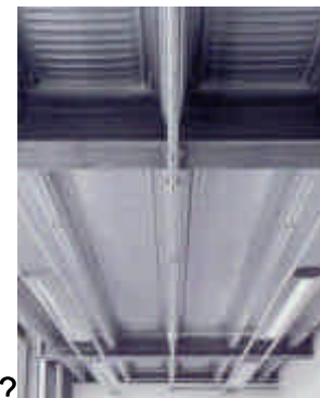
Impressions from the building process and from the decking system HOESCH Additiv Decke
