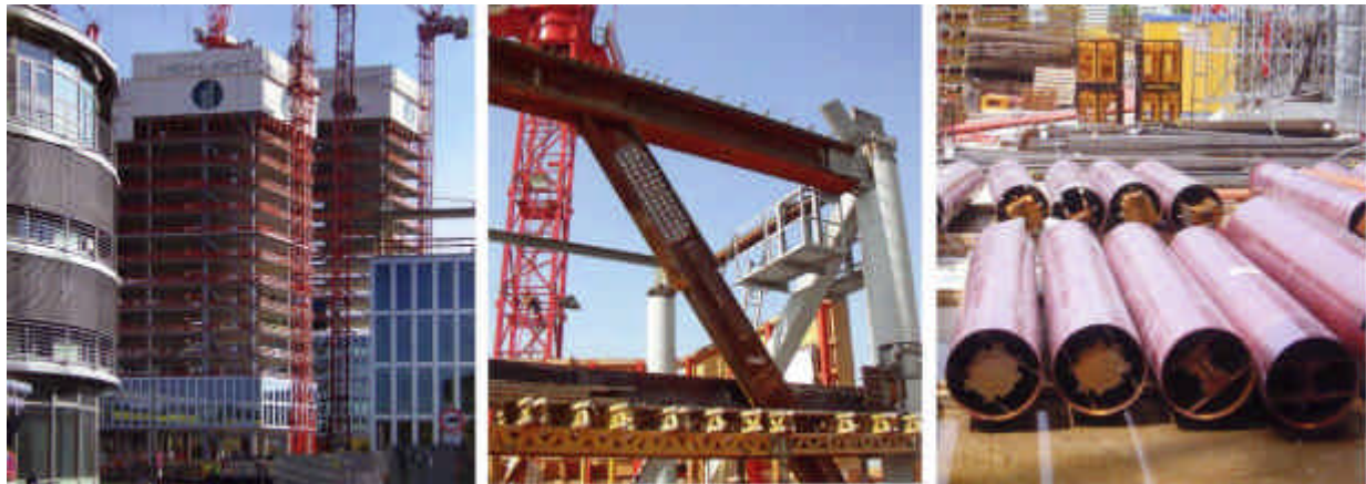
Impressions from the construction process of the steel framework bracings, [2]
