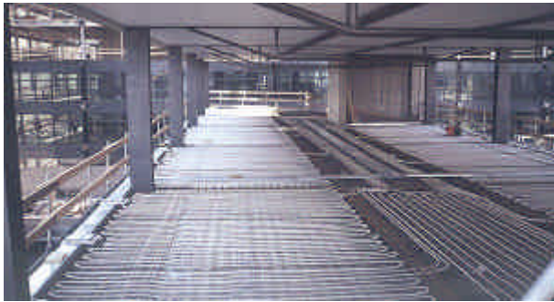
Water heating/cooling pipework laid within the floor slab
