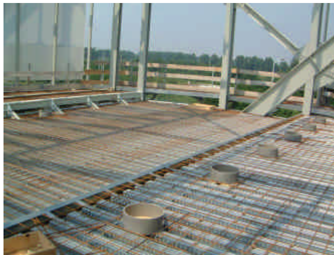
Composite slab used in the auditorium area
