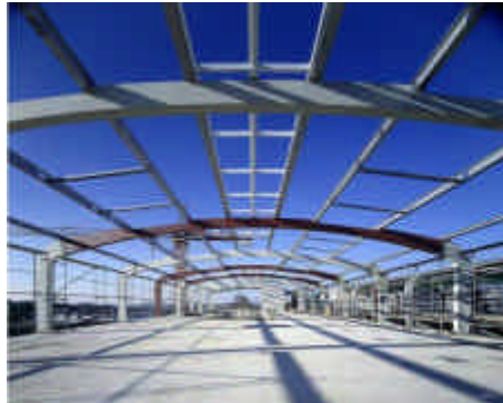
Office level under construction
