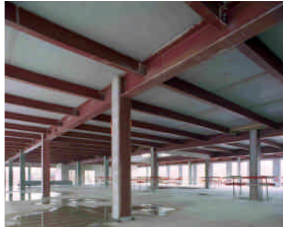
Main and secondary beams with partially encased columns
