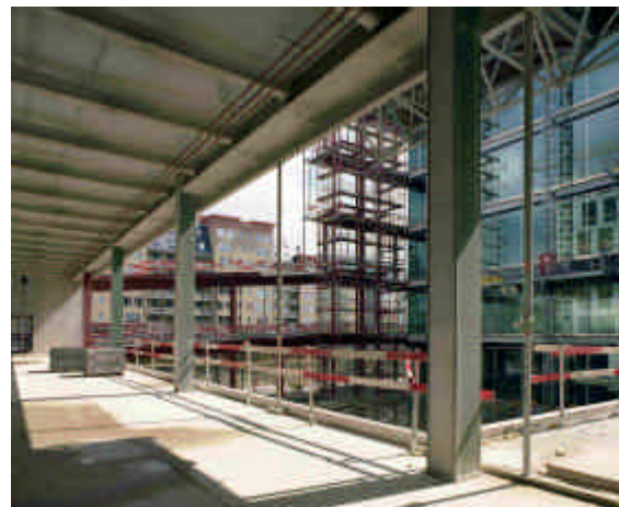
Spray fire protection
