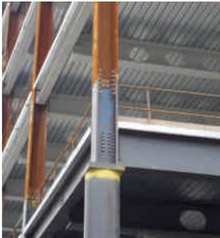
Detail of tubular construction
