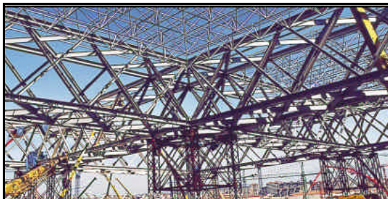
Hall structure during erection
